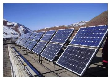
Figure 3: mono-crystalline silicon solar panels [6]
